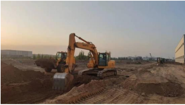
Figure 5. Airport construction experiments.
